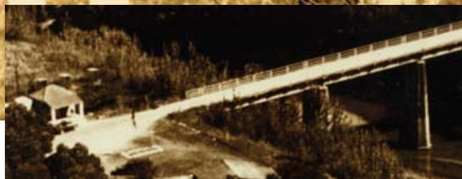
Caledon River Bridge
